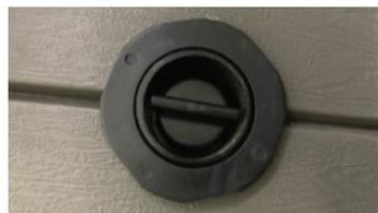
Your drain valve will look something like this. To operate, unscrew the center section and screw in the drain valve adapter that arrived with your hot tub. The action of screwing in the drain valve adapter releases the water flow.
